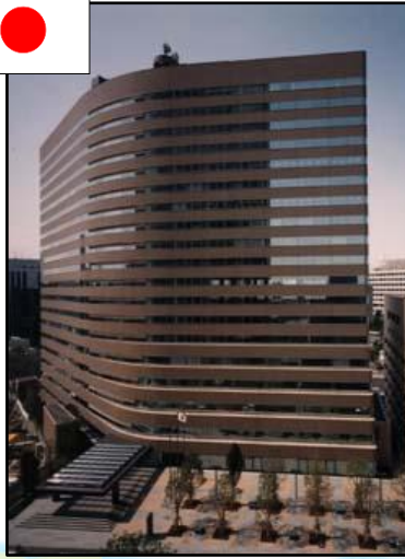
PMDA Central Office, Tokyo
