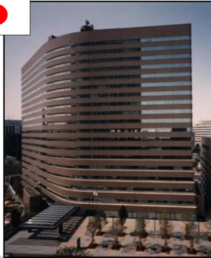
PMDA Central Office, Tokyo
