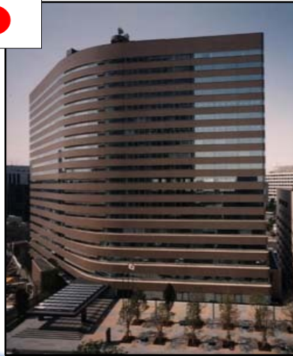
PMDA Central Office, Tokyo
